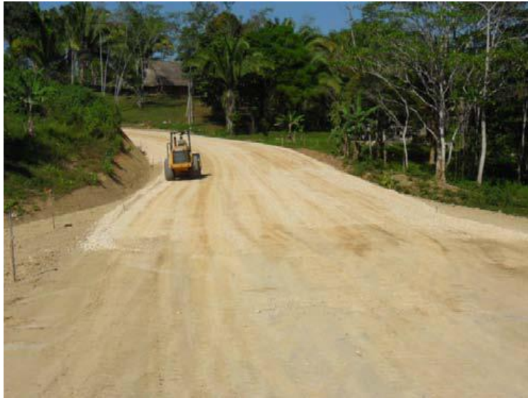
Photo 3: Sub- base being compacted- Ch 25100m
