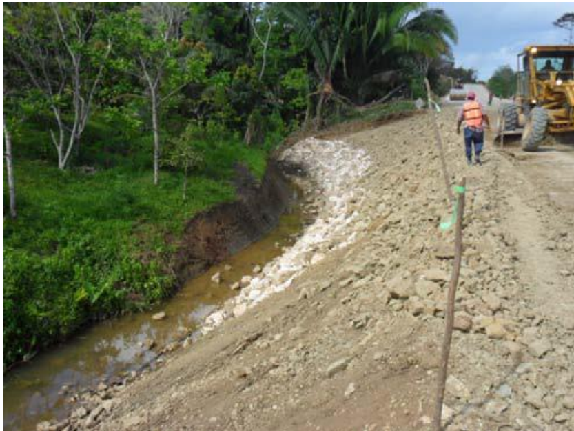
Photo 4: Rip placed for embankment toe protection- Ch 24700m.
