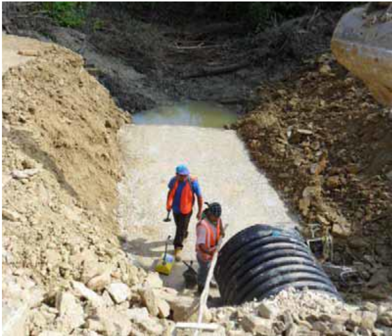
Photo 5: Culvert installation at Ch 28960m.
