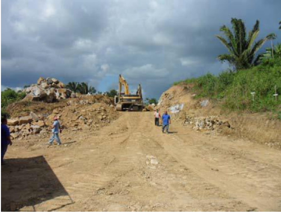
Photo 1: Cut site 28320m – 38400m. Excavator and rock breaker working.
