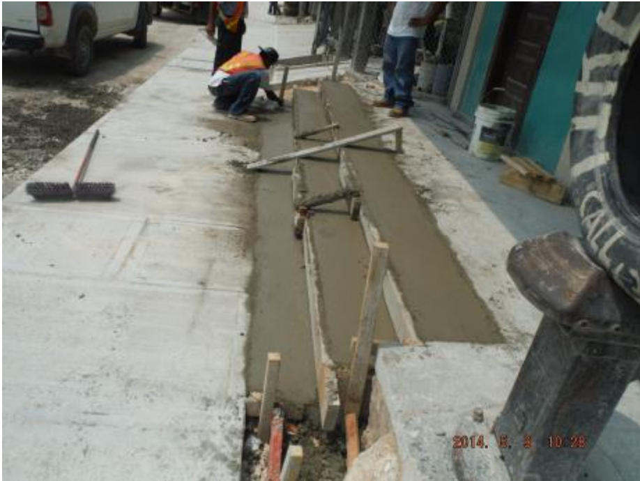
Photo 5: Joseph Andrews- Accommodation Works
