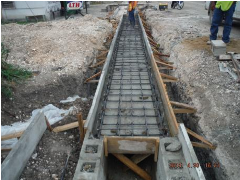
Photo 6: Joseph Andrew- Box Drain Construction
