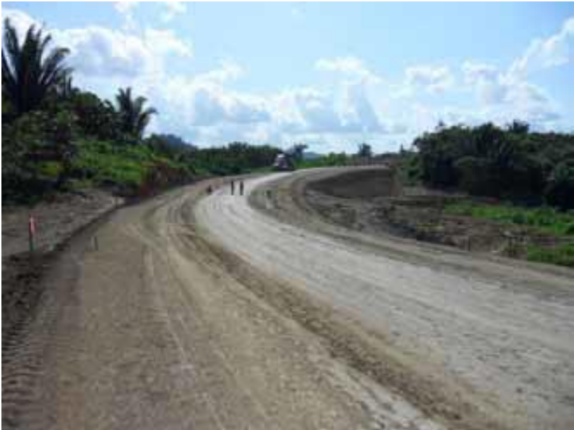
Photo 3: Subgrade nearing completion Ch 28500m (approx.)
