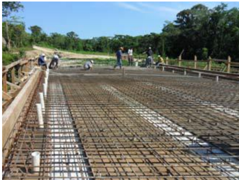
Photo 6: -Rio Blanco Bridge - placing deck steel.
