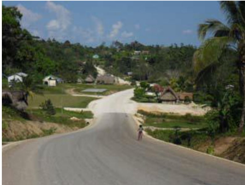
Photo 5: Extention of 1 st coat seal into Santa Elena Village.
