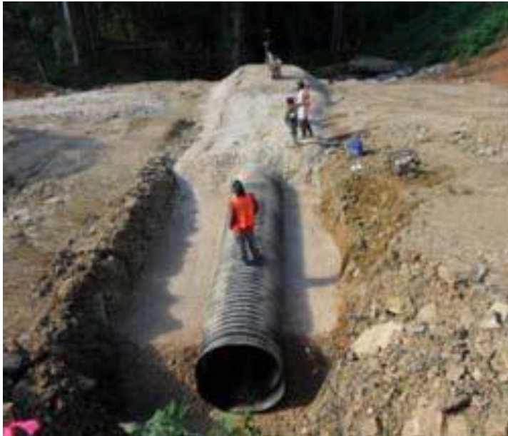
Photo 1: Culvert being installed at chainage 28350m
