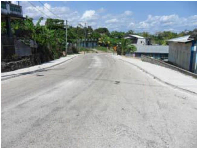
Photo 4: San Antonio Village- 1 st coat seal and concrete footpaths.
