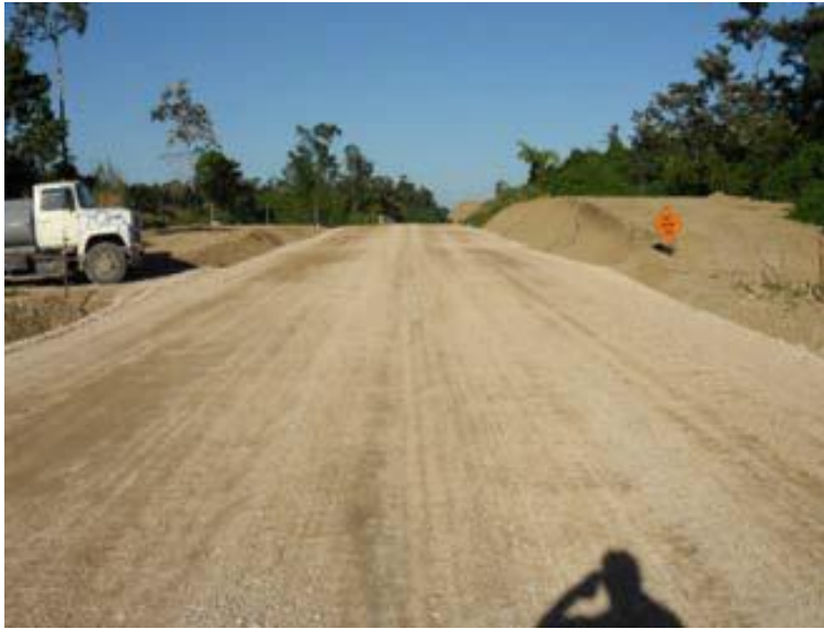
Photo 3: Subgrade preparation at approx Ch24400m
