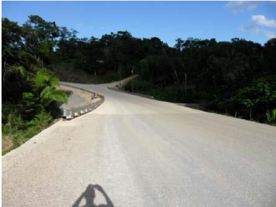
Photo 5: Guardrail being installed at Ch 11400m (San Antonio Village).
